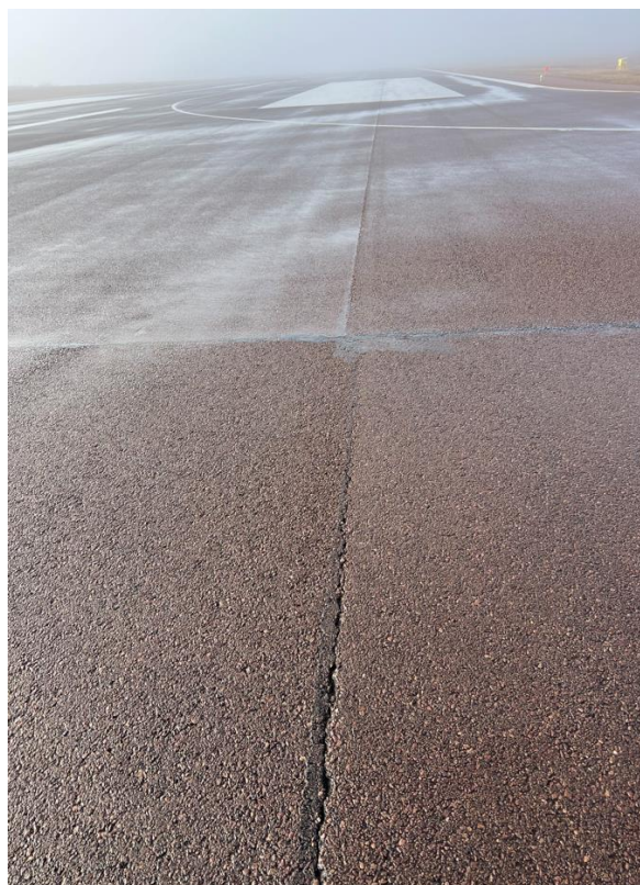
Fissure de joint
