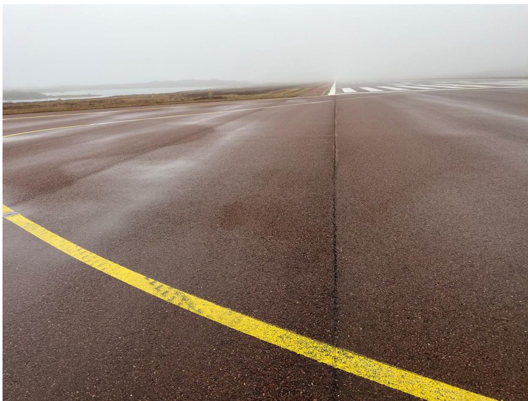
Fissures de joint
